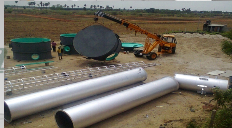
ANGLO FRENCH TEXTILES MILL CHIMNEY ERECTION WORK
