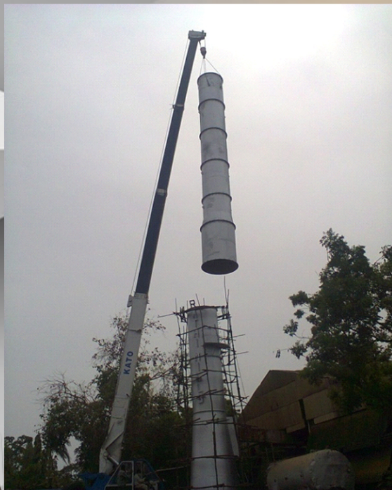
ANGLO FRENCH TEXTILES MILL CHIMNEY ERECTION WORK.
